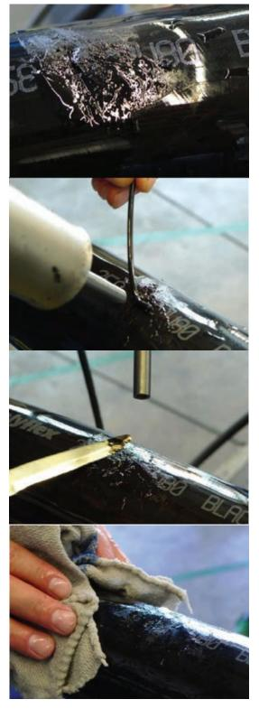
Appendix 3: Procedure for a repair of a local damage in the outer cover
